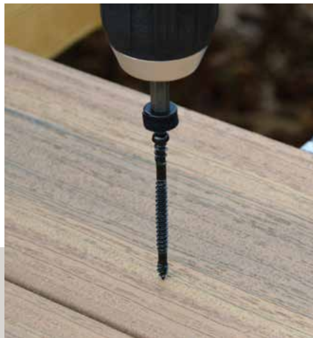
A special driving tip automatically puts the screw at a precise depth.
