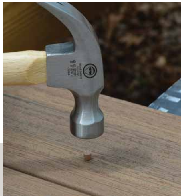
Then, the color-matched plug is tapped in with a hammer.
